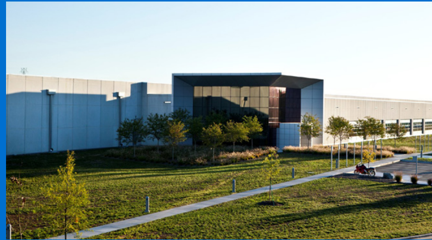
LEED New Construction Gold Certified data center in North Carolina
