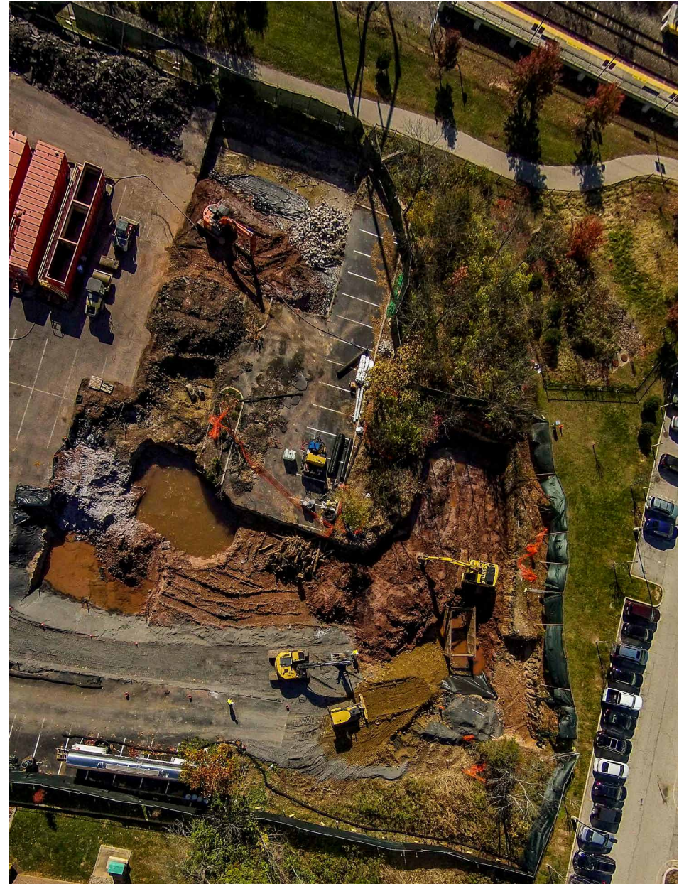
Manufactured gas plant remediation in progress, southeastern Pennsylvania.
