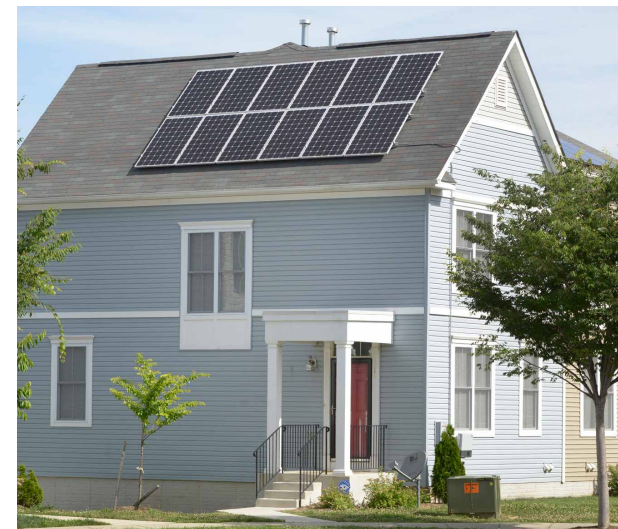
Exelon enables distributed energy integration into the grid of the future.
