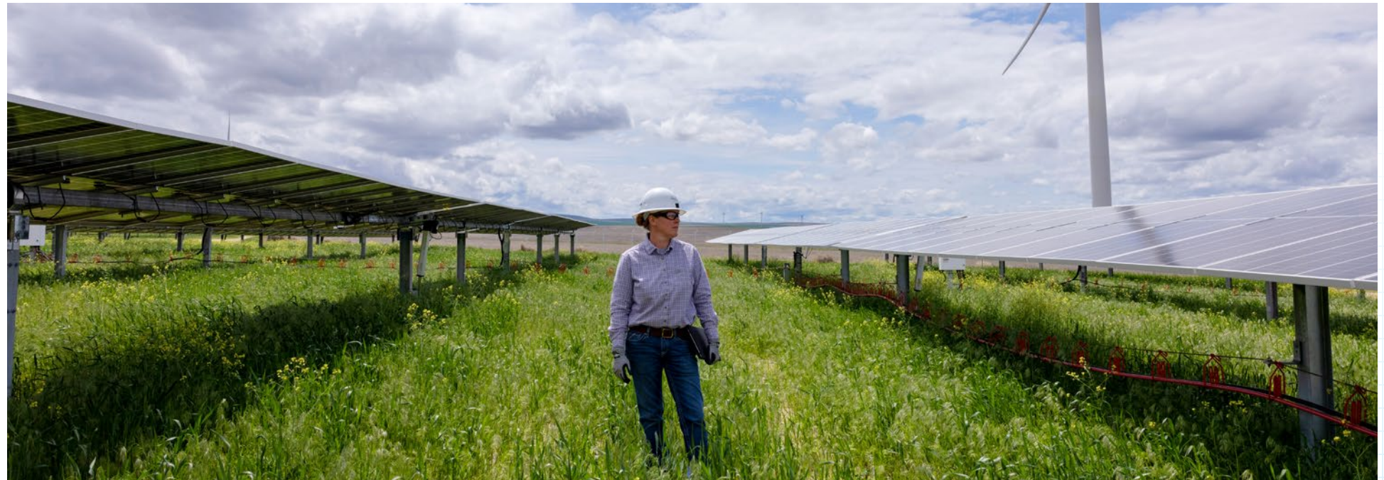
Employee Jana Lehn surveys solar panels at the Wheatridge Renewable Energy Facility in Lexington, Ore. The operation combines solar with wind and battery storage.
