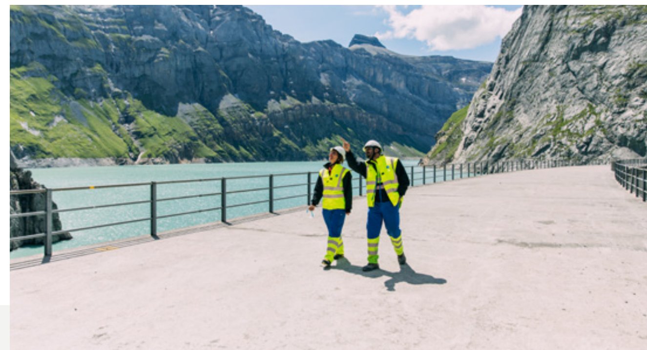
Hydro power stations, Linthal, Switzerland
