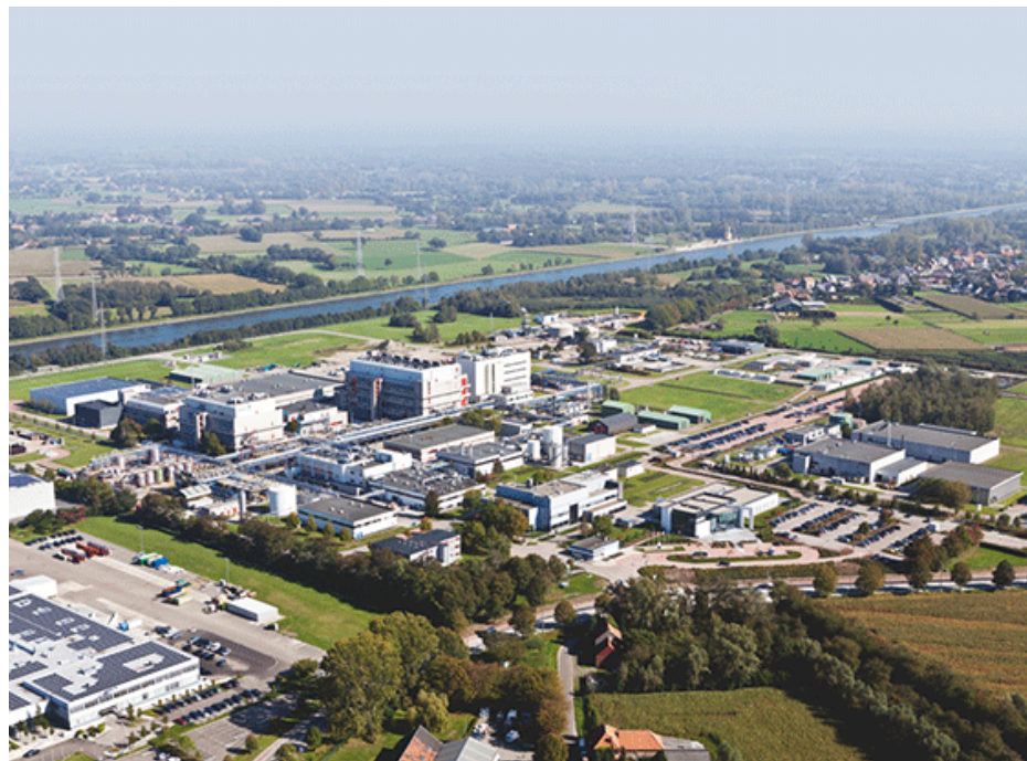
Our Geel, Belgium, site.
