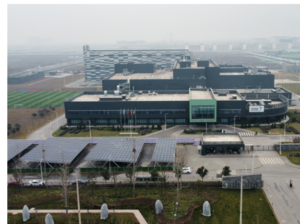
Our LEED Gold-certified Xi'an, China, Janssen facility with a 1 MW solar array installed in 2020.
