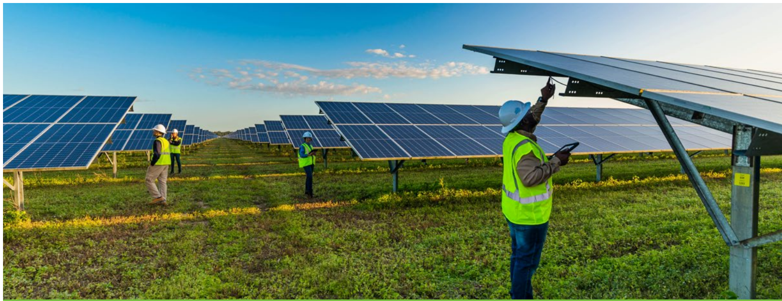
Crews work to commission the FPL Miami-Dade Solar Energy Center in Miami-Dade County Florida.
