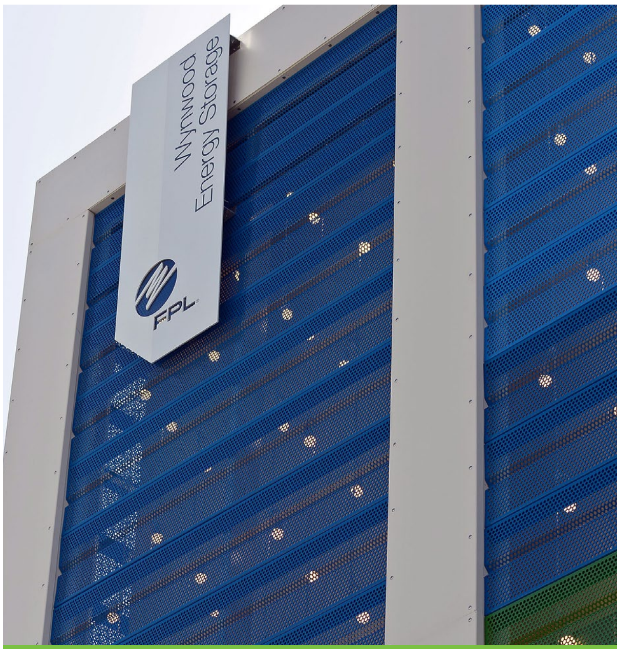
FPL Wynwood Energy Storage in Miami, Florida.
