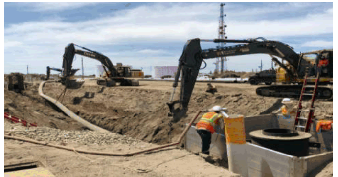
Crews work on a new industrial wastewater system in JR Davis Yard.
