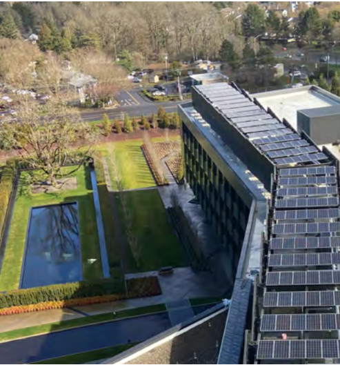
Solar panels on Serena Building, NIKE WHQ – Beaverton, OR
